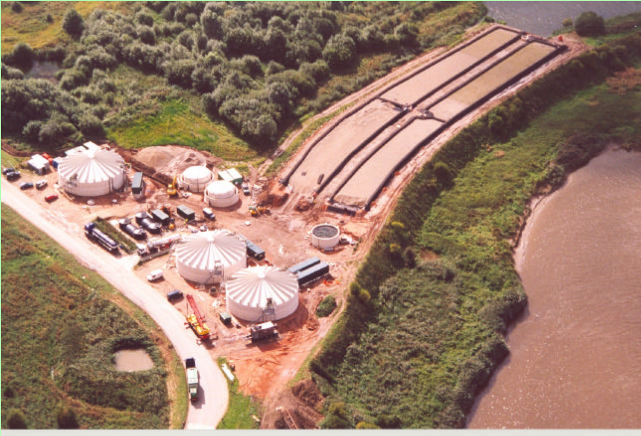
Plant under construction, showing the twin row leachate balancing tanks, three large SBR tanks, and effluent balance tank and reed beds top right (Robinson, Sardinia 2003)
