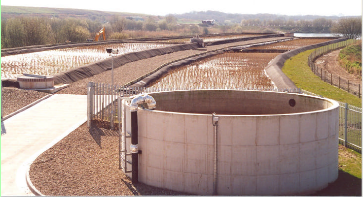
Effluent balance tank, and recently planted reed beds (Robinson, Proceedings Sardinia 2003)
